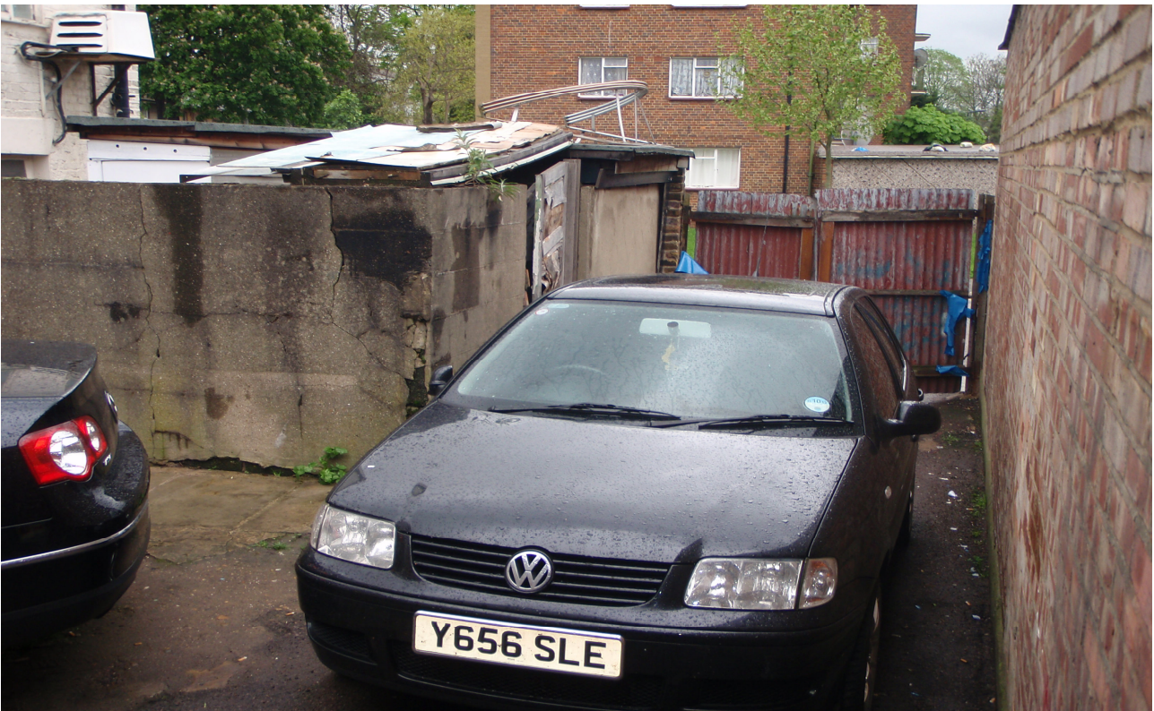
The emergency door opens onto this car park, which belongs to the next door shop. Emergency exit is via the two gates at the end of the car park. This area is NOT to be used for smoking. Smokers are to be directed to the street at the front entrance of the premises.
