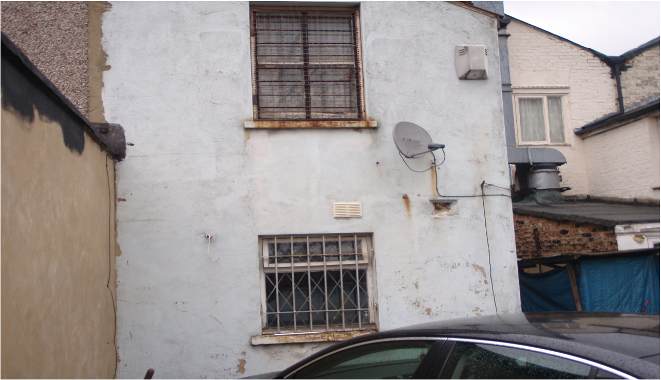
Rear of next door shop premises. It appears that the first floor is not residential.
