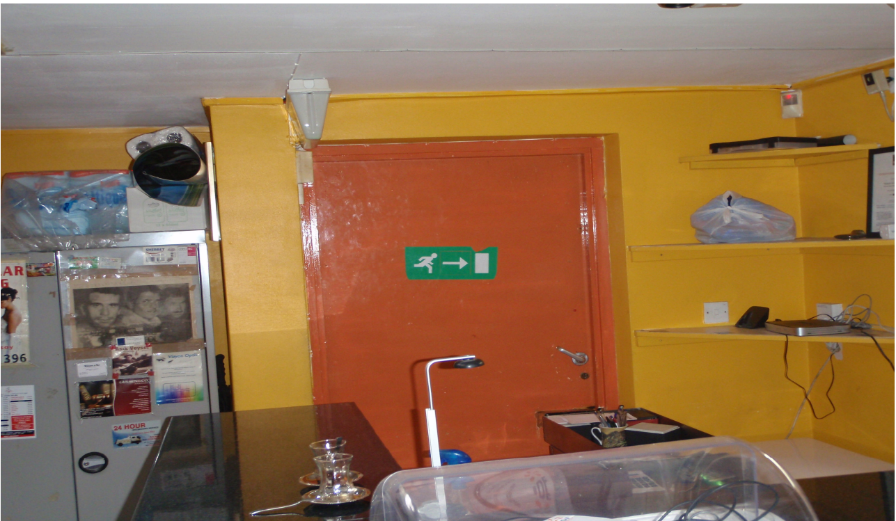
This is the fire exit door at the rear of the room behind the counter. It is intended that this is not used by the public unless in an emergency. The door to remain closed at all times, apart from the occasional use by staff.
