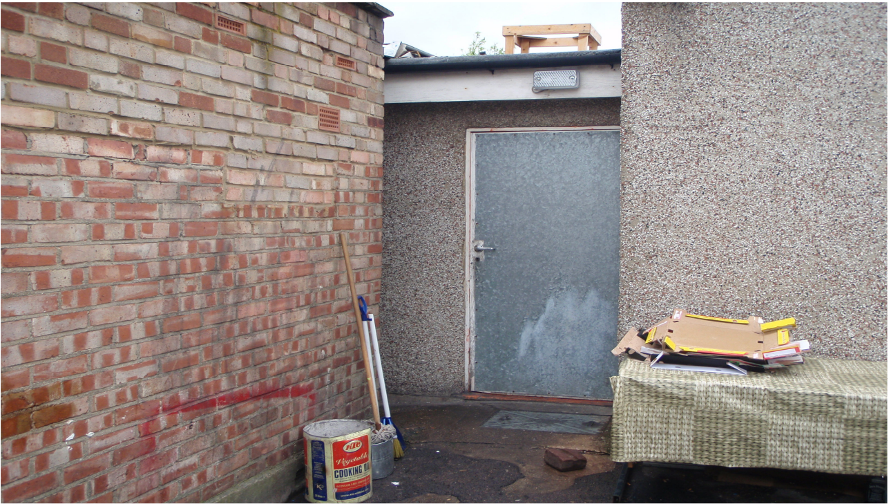
View from outside the rear emergency door.
